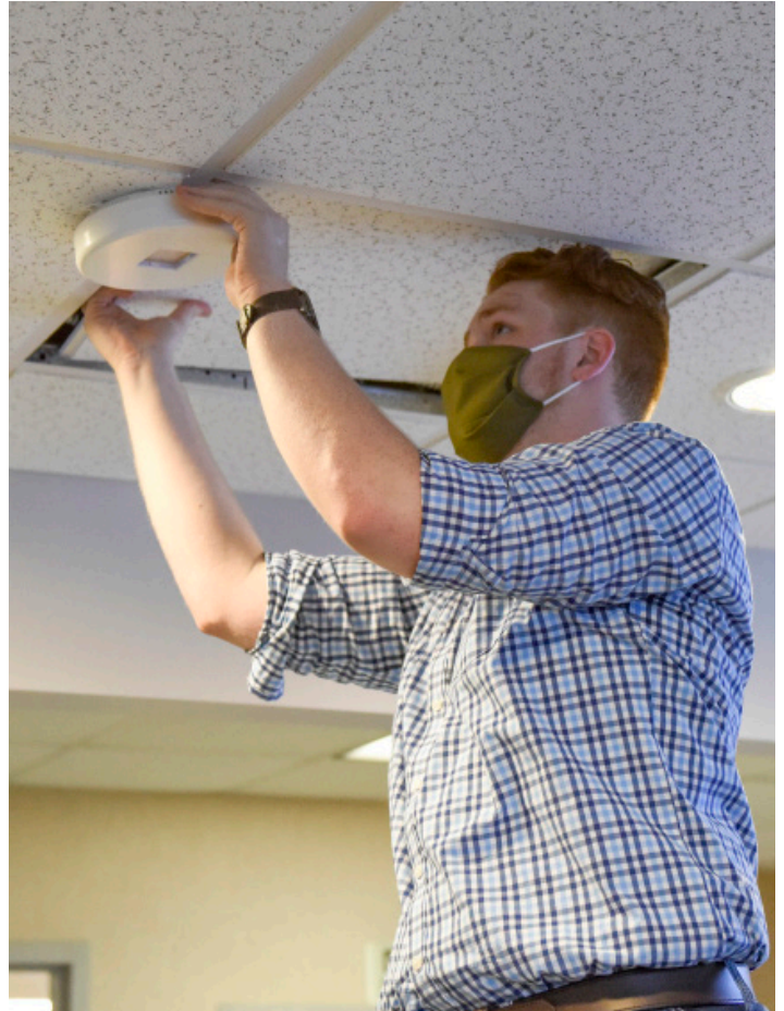
Jordan, a field engineer for FAR UV Technologies, installs an ultraviolet light in the 189th Operations Group ceiling July 16, 2020, at Little Rock Air Force Base, Ark. The UV lighting is environmentally-friendly and mercury-free. (U.S. Air National Guard photo by Master Sgt. Jessica Roles)
