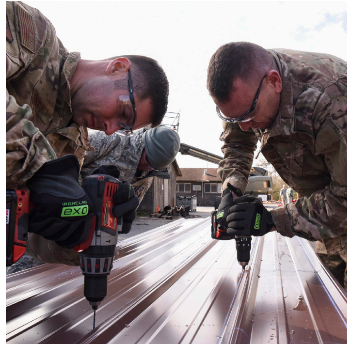
MSgt. David Foret and Senior Master Sgt. Kevin Bright, both assigned to the 189th Civil Engineering Squadron, drill holes into metal roofing to prepare it for installation at Little Rock Air Force Base, Ark. on February 26, 2019. The 189th and 19th CES are working together to revitalize the base’s deployment readiness training grounds.
