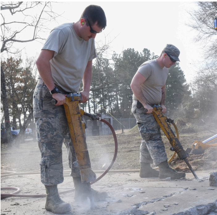
Two Airmen from the 19th Civil Engineering Squadron use jackhammers to break a concrete slab at Camp Warlord at Little Rock Air Force Base, Ark. on February 26, 2019. Airmen from the 189th and 19th CES are working collectively to revitalize the base’s deployment readiness training area. (U.S. Air National Guard photos by Senior Airman Kayla K. Edwards)
